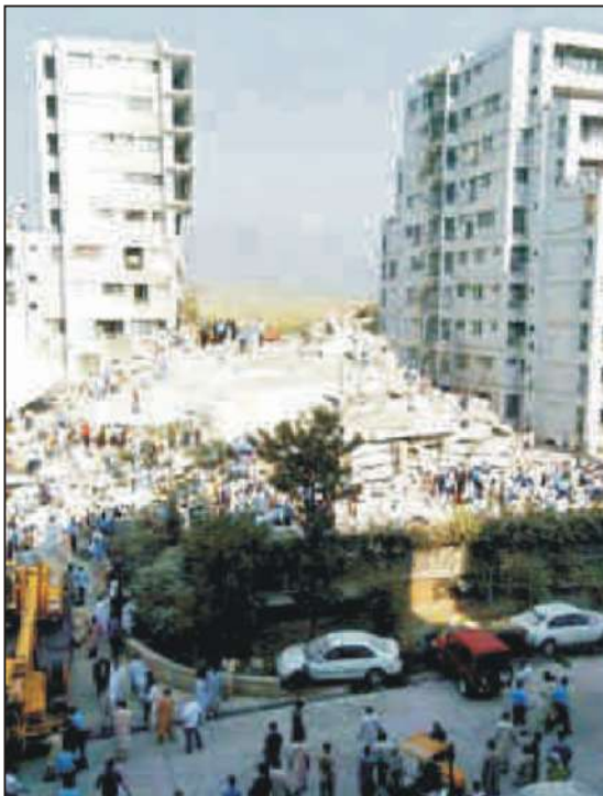
Fig 1.3: Margala Tower Islamabad collapsed during October 2005 earthquake
