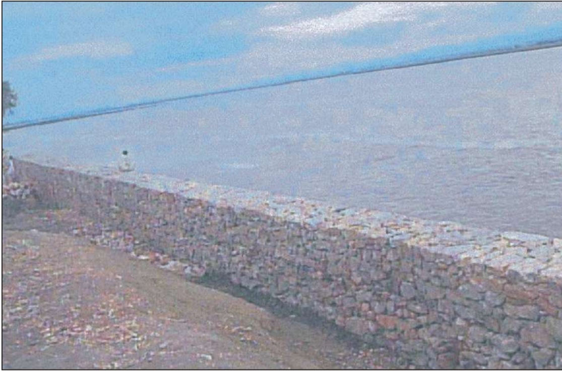
Fig. 3.5 and 3.6: Flood mitigation measures (Structural adjustment)
