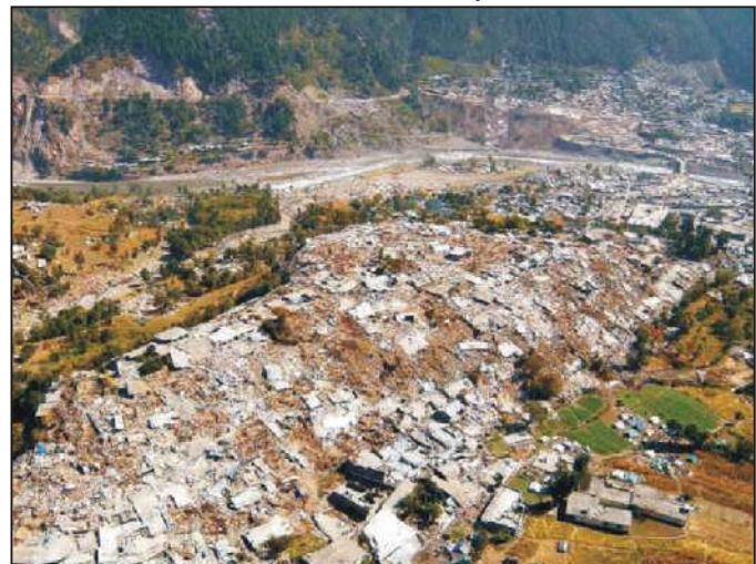
Fig 1.1: Balakot City devastaion during October 2005 earthquake
